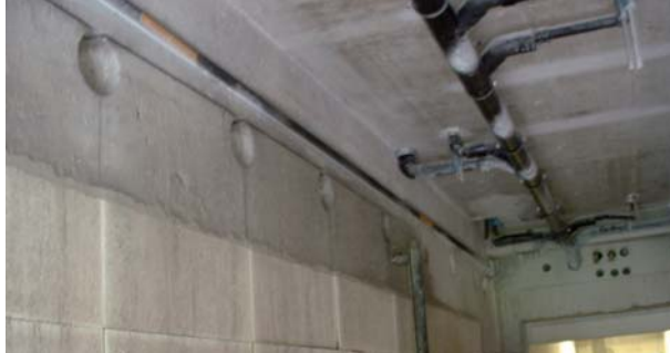
Wall after cutting into 1 m 2 sections
