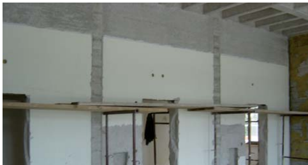
The room before the start of the works
