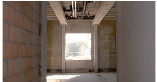
Completion of the works with the walls removed
