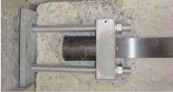
End anchor in the building isolation joint
