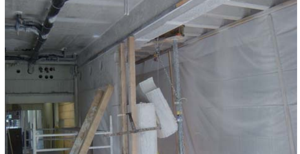
Removing the cut concrete sections
