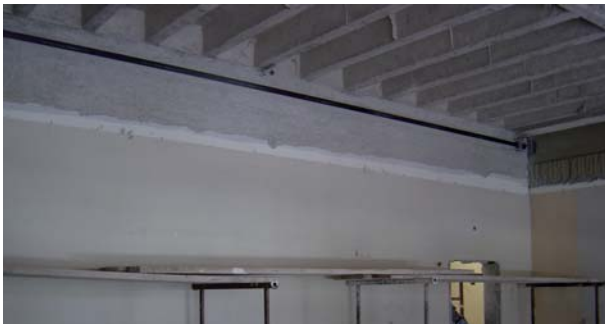
Room A during post-tensioning works
