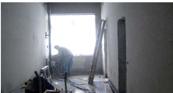
Cutting the vertical slots
