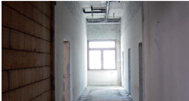
Walls before the start of the works
