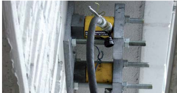
Post-tensioning jacks in operation
