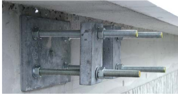
End anchor on the outside of the building
