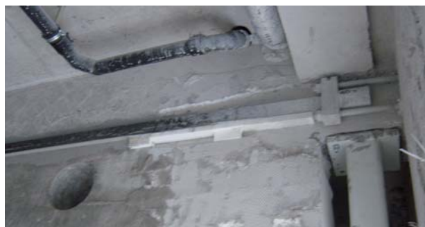
Steel support installed on the outside wall
